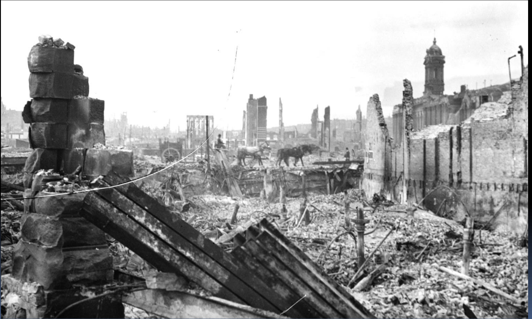
Aftermath of the 1906 earthquake
